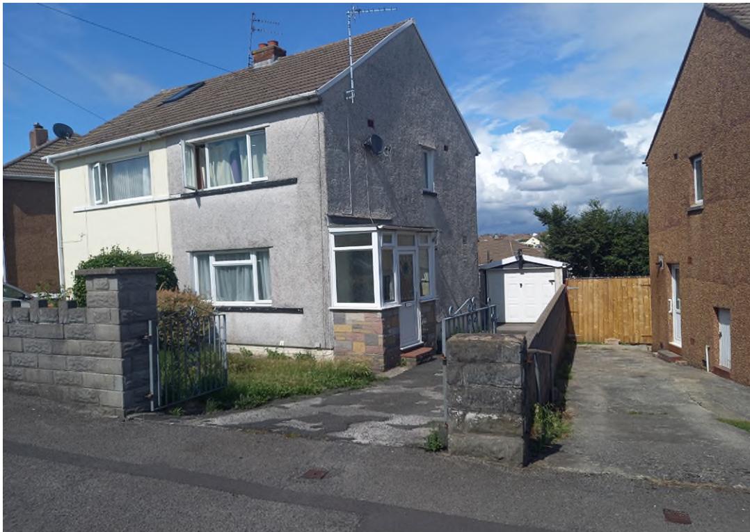
Figure 1 - Photograph of Existing Property:
